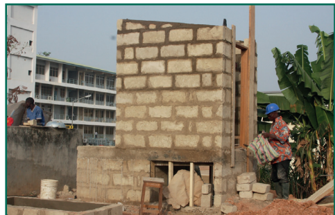
Figure 47 Constructing the superstructure
