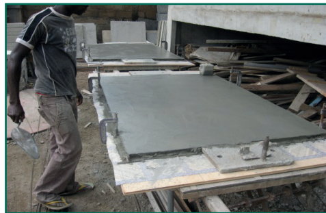
Figure 63 Finishing the pre-cast slab
