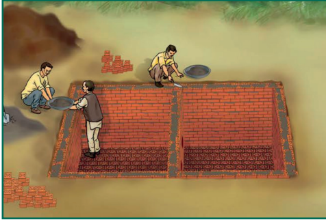
Figure 56 Constructing the tanks/chambers
