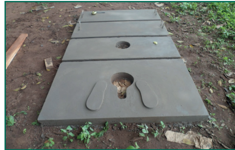
Figure 35 Casted slabs
