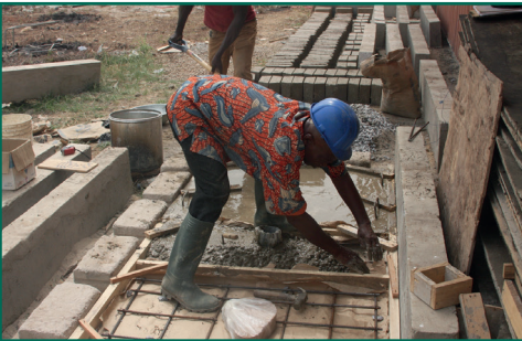
Figure 34 Casting the cover slabs
