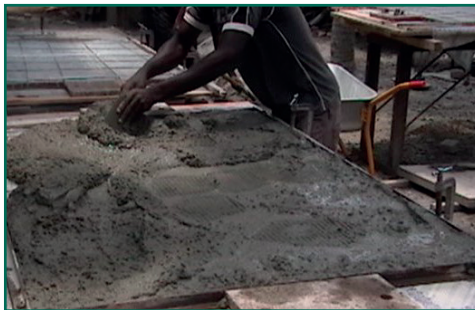
Figure 62 Spreading of mortar on formwork
