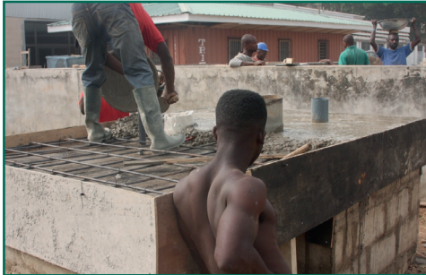
Figure 45 Decking of the vault
