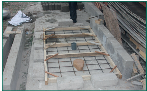
Figure 33 Preparing framework for reinforced cover slab
