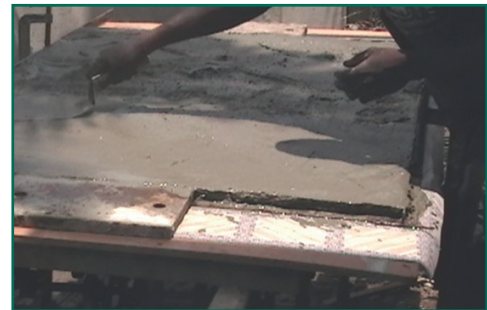
Figure 62 Spreading of mortar on formwork
