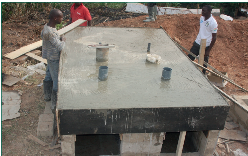
Figure 46 A fully decked UDDT vault
