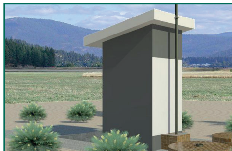
Figure 15 Back view of a pour-flush toilet
