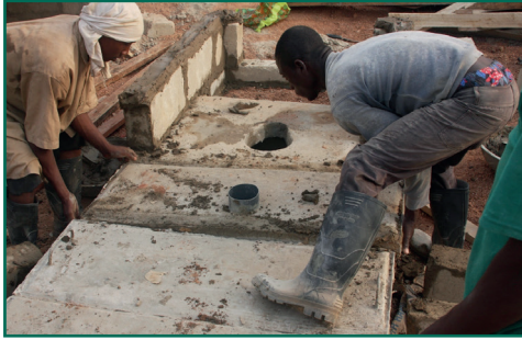
Figure 36 Placing the slabs on pit
