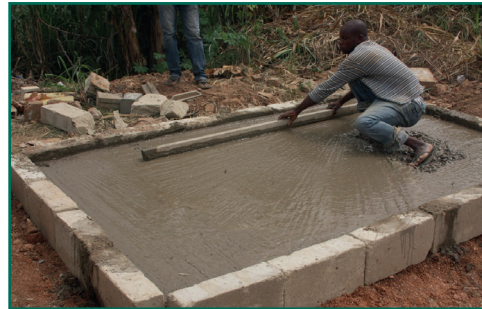
Figure 42 Dressing the foundation
