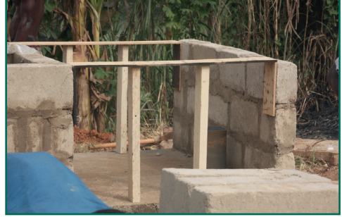
Figure 44 Preparing for decking of the vault
