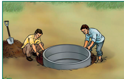
Figure 51 Pit being lined with ring concrete
