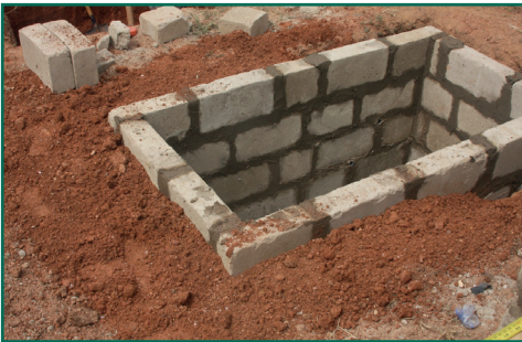
Figure 32 A rectangular pit lined with blocks
