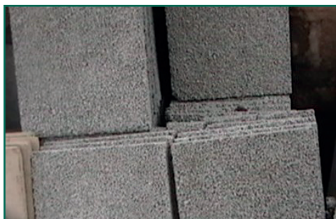
Figure 64 Pre-cast porous concrete
