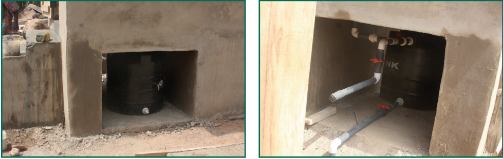
Figure 48 Installing the urine storage tank
