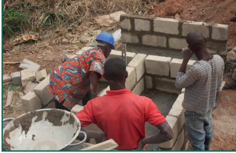
Figure 43 Constructing the vault
