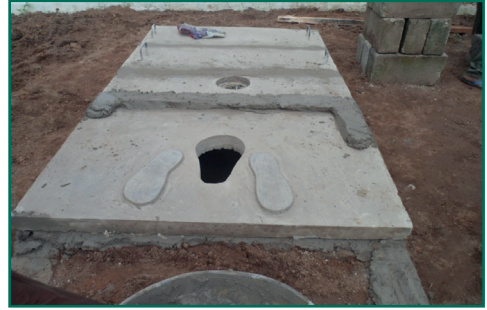
Figure 37 Slabs secured on pit
