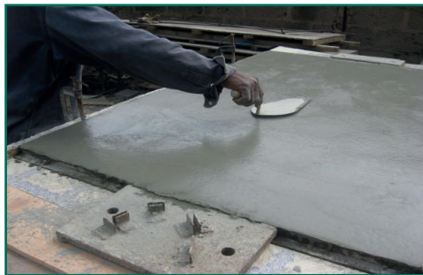
Figure 63 Finishing the pre-cast slab
