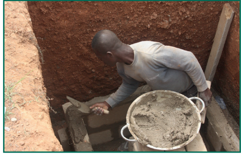
Figure 31 Digging and lining of pit
