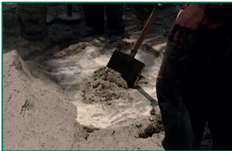
Figure 61 Mixing of concrete and mortar
