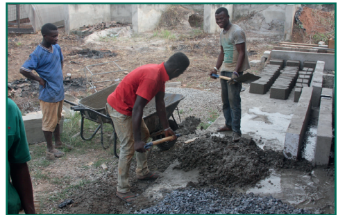
Figure 61 Mixing of concrete and mortar
