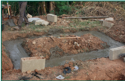
Figure 41 Preparing the UDDT foundation
