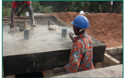
Figure 45 Decking of the vault
