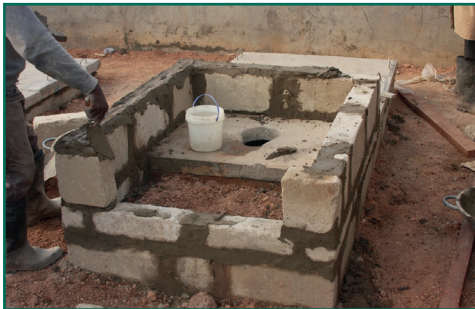
Figure 38 Building the superstructure
