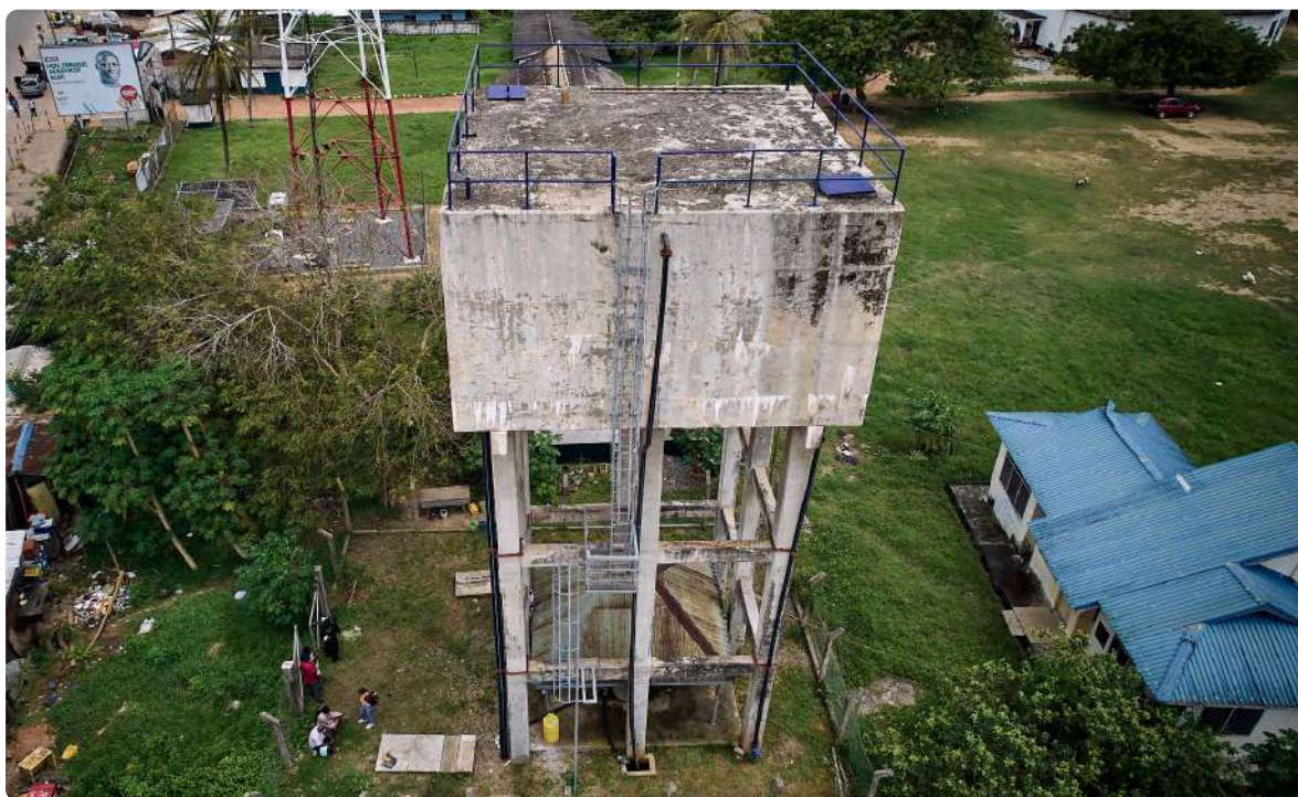
New ladder at the Esiamia water system, installed by Safe Water Network
